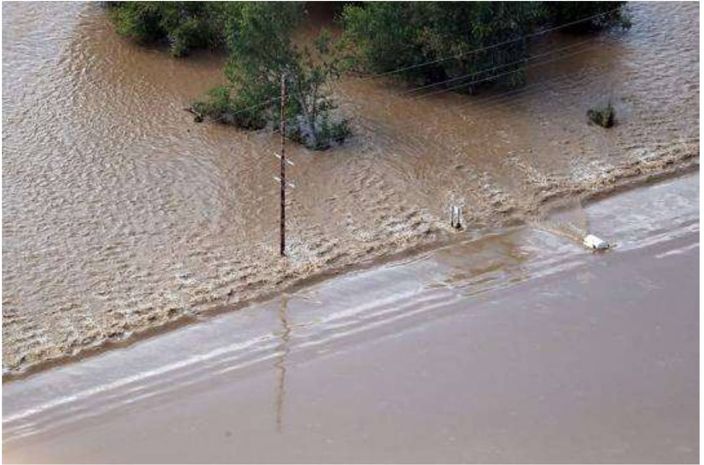
Water flows over Hwy. 56 near Viola on Wednesday, Aug. 29.
