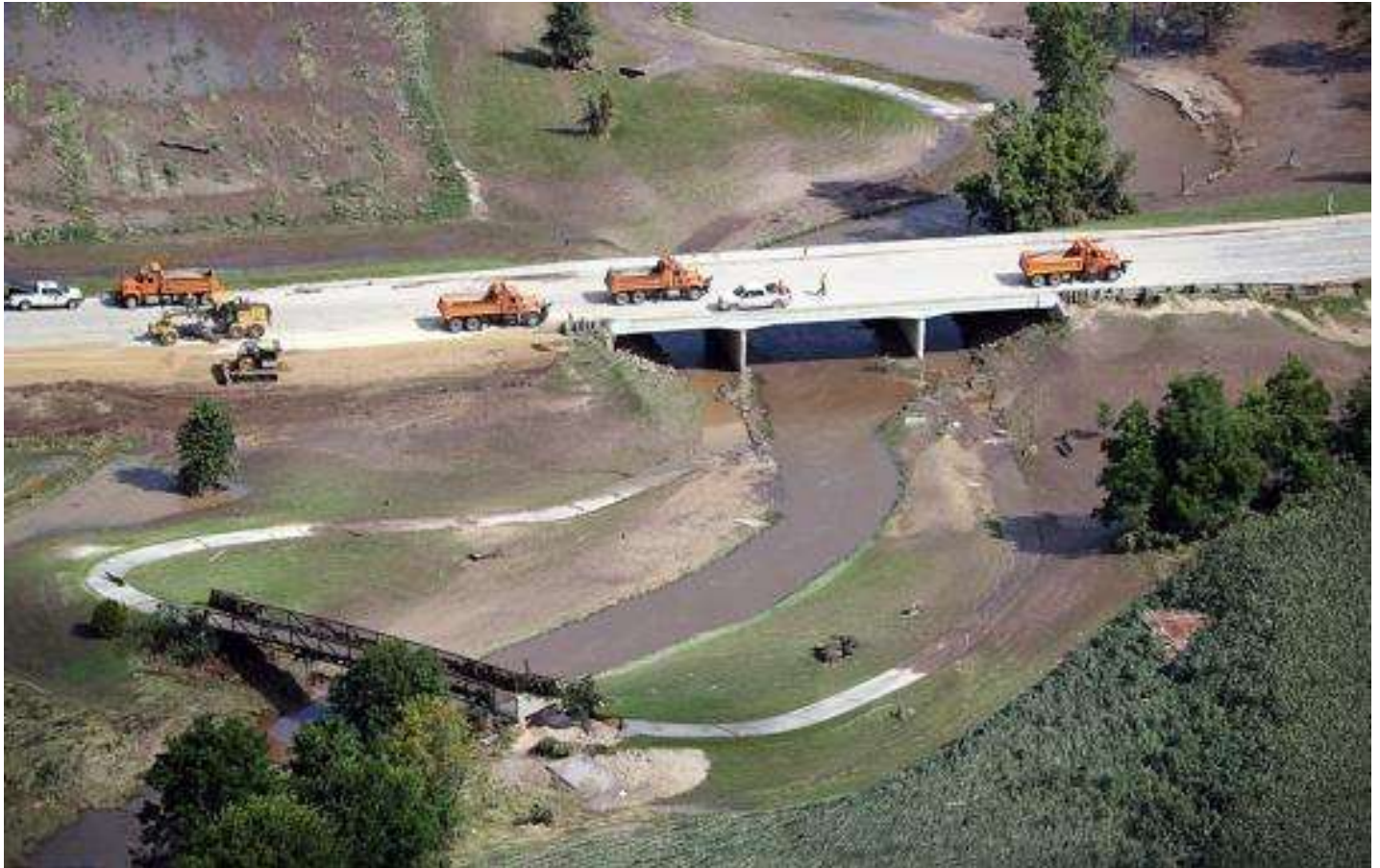
The 14/61 bridge in Coon Valley on Wednesday, Aug. 29.
