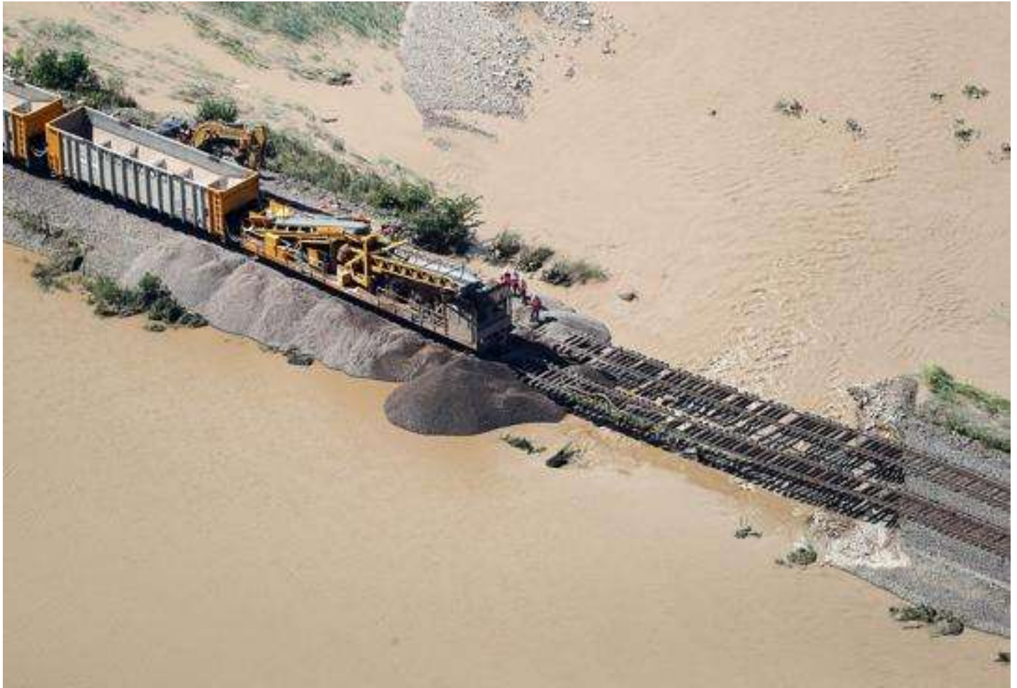
Crews work to repair railroad tracks near Stoddard on Wednesday.
