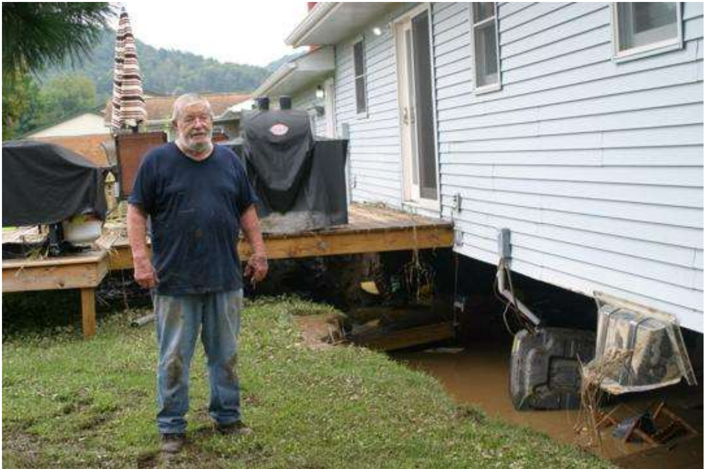
Richard Mixer of Coon Valley is missing the entire back wall of his basement after it was blown out by flood waters. Dorothy Robson, Westby Times
